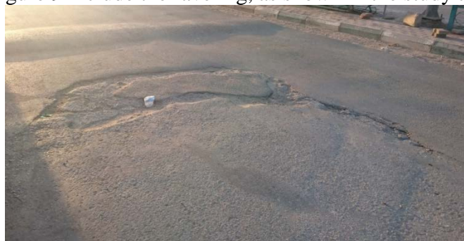
Figure 9 Raveling, corrugation and longitudinal crack distresses in study area
