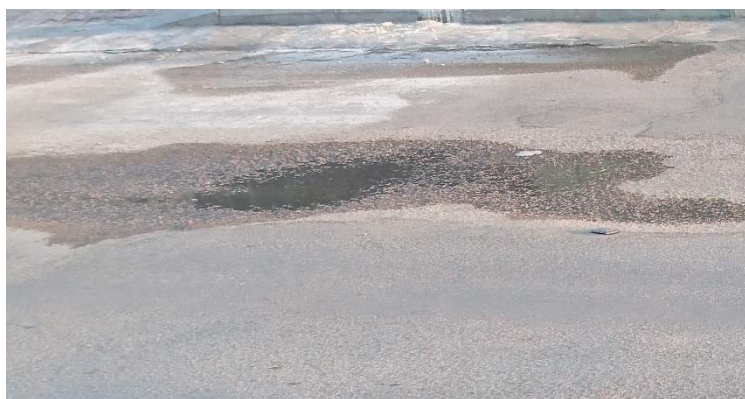
Figure 11 Depression distresses filled with water
