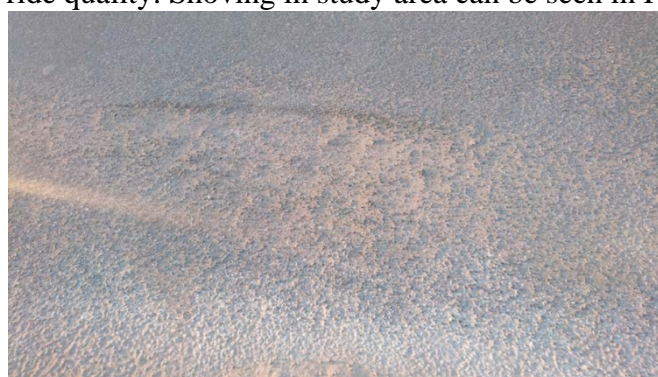
Figure 10 weathering and polished aggregate distress in study area
