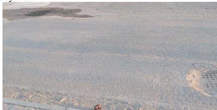
Figure 8 Rutting and depression distresses in study area
