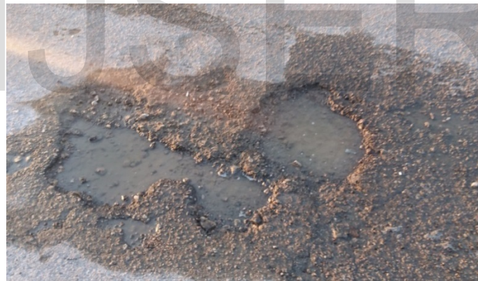
Figure 7 Pothole distress in study area
