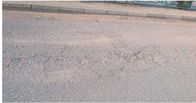
Figure 5 Alligator crack distress in study area
